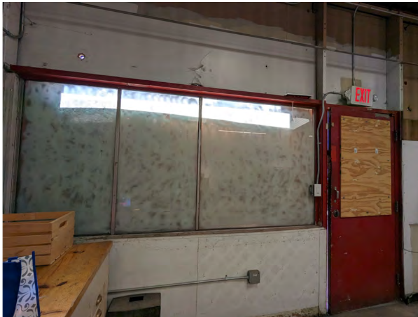
Figure 5- Boarded up glass windows and doors in the existing Primary Warehouse.
