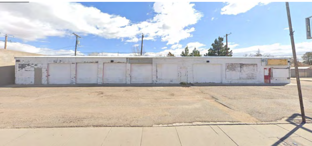
View of existing unused warehouse building to be remodeled and expanded.
