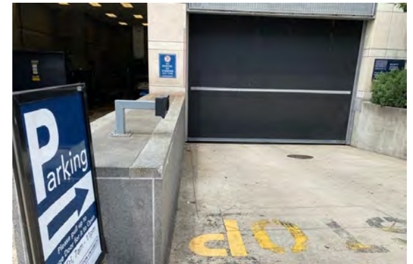
Sealed Parking Garage Requiring Access Code or Key Card in Washington, DC
