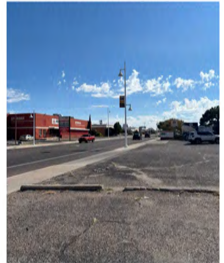
Uneven/cracked parking surface
