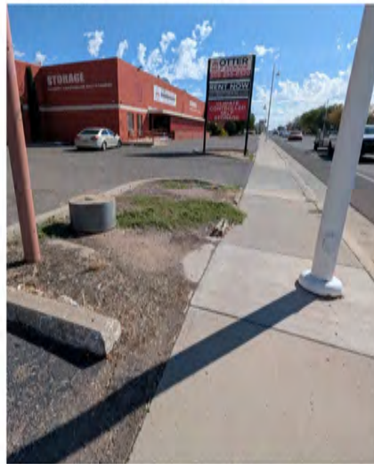
Damaged pavement surface
