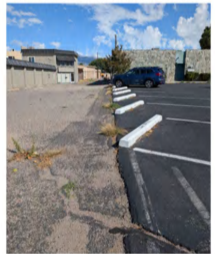
Uneven/cracked parking surfaces
