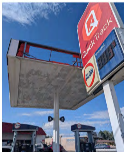
Damaged roof
