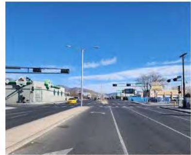
FIGURE 68. Central Ave & Pennsylvania Ave looking East
