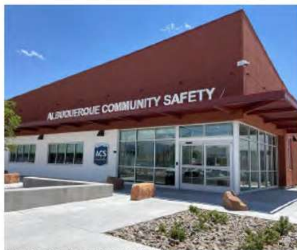
FIGURE 64. ACS at San Mateo Blvd
