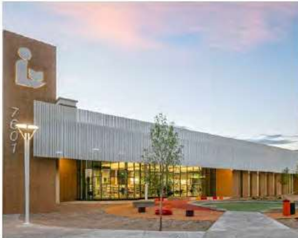
FIGURE 6. CABQ International Library (Source: RNKM Architecture)
