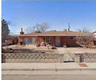
FIGURE 59. Single Family Residence
