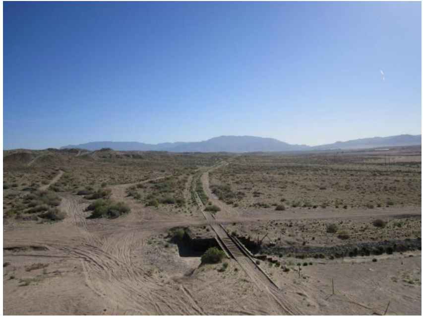
Figure 5 The Unused Portion of the Spur Is in Disrepair
