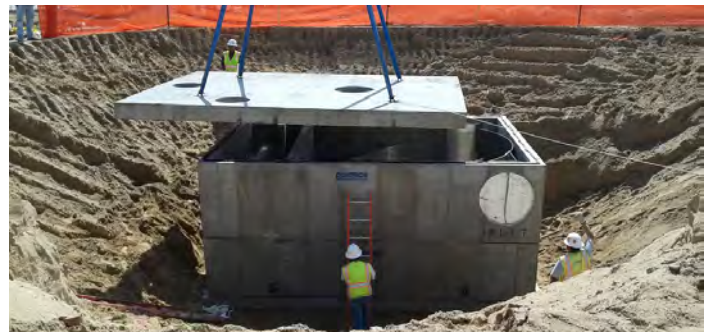
WSP designed a water quality structure for treating on-site storm water specifically to fit the unique needs of the Daytona Transit Facility project for the City.
