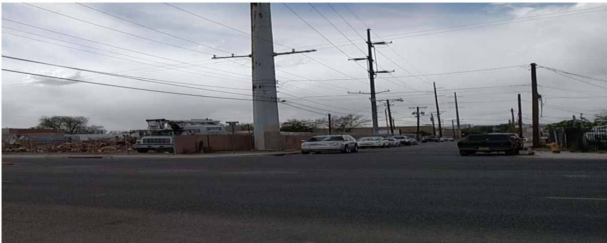
Major overhead transmission lines with poles in the middle of sidewalks.
