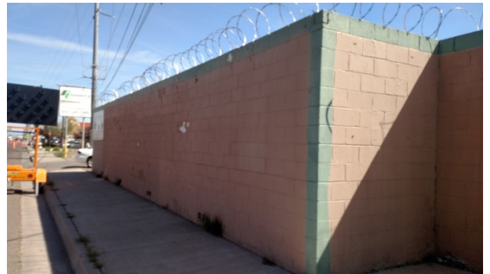
Blank wall topped with razor wire
