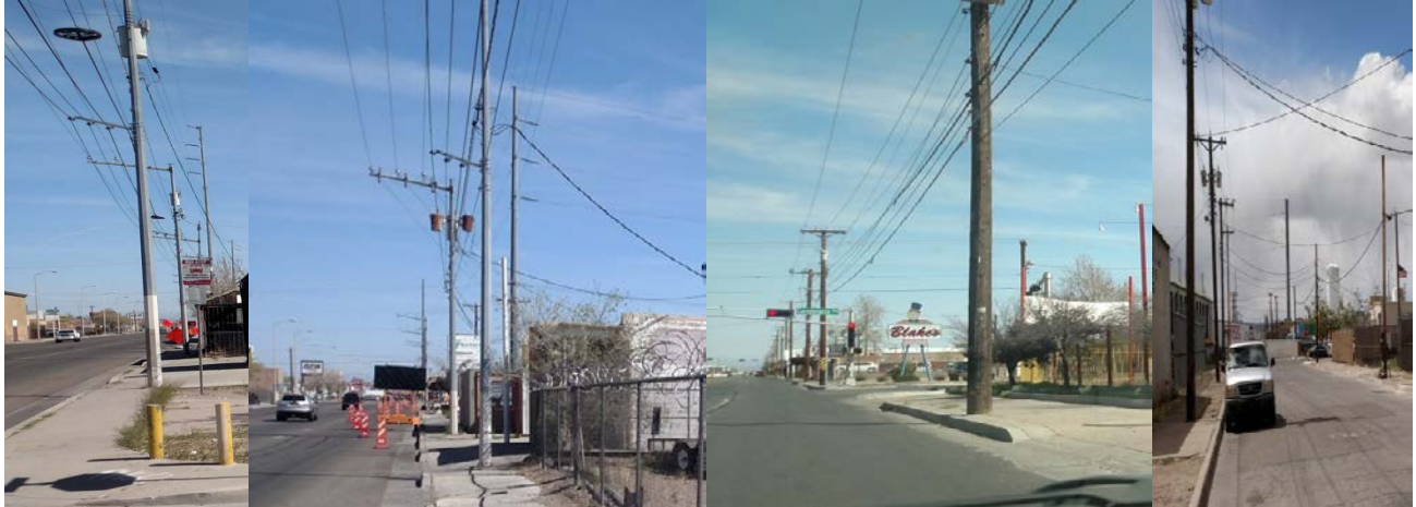
Various overhead power lines that are common throughout this area.
