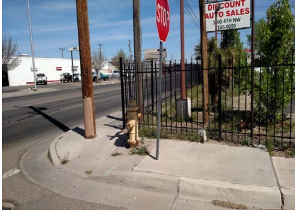
Numerous obstructions in the sidewalk
