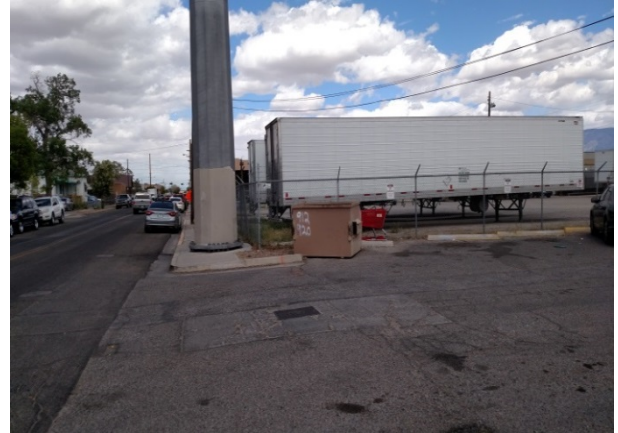
Large power-pole in the sidewalk
