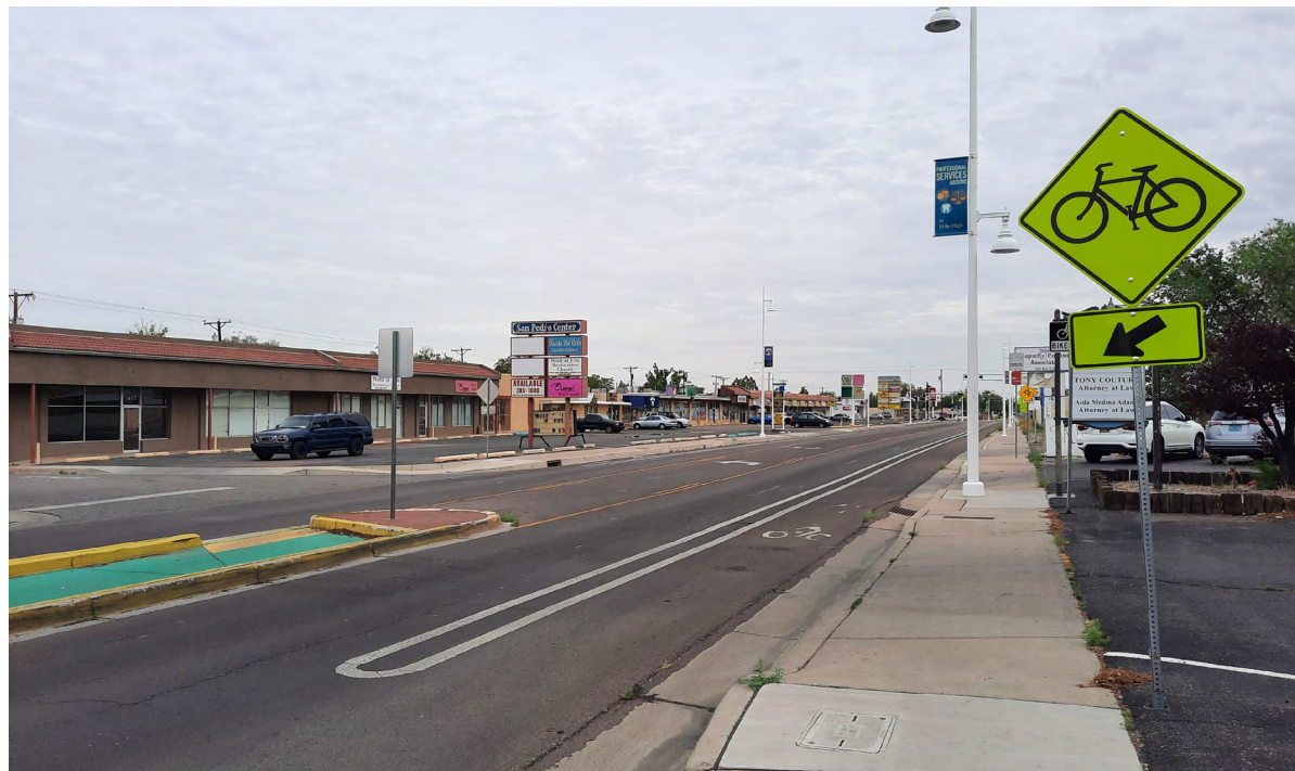
The City installed buffered bike lanes along San Pedro Drive as part of a road diet in which one lane of traffic was removed in each direction to reduce travel speeds and create safer conditions for people walking and biking.
