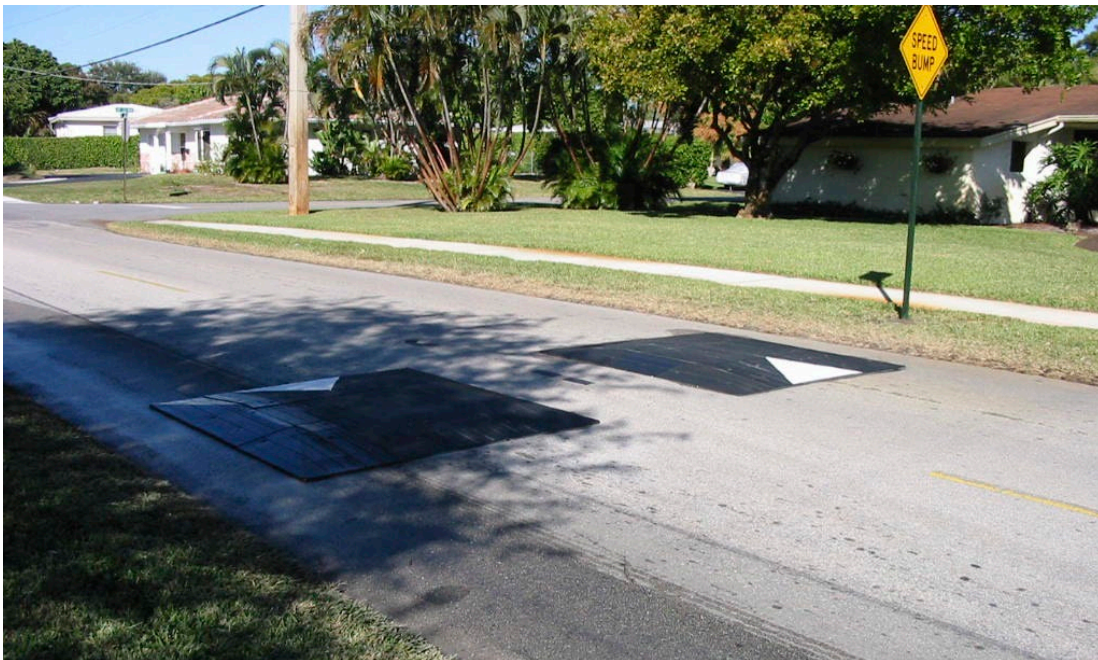
Figure 21: Example of Speed Cushion
