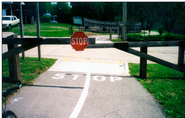
Figure 5-21: Gates across a bicycle path (not recommended)
