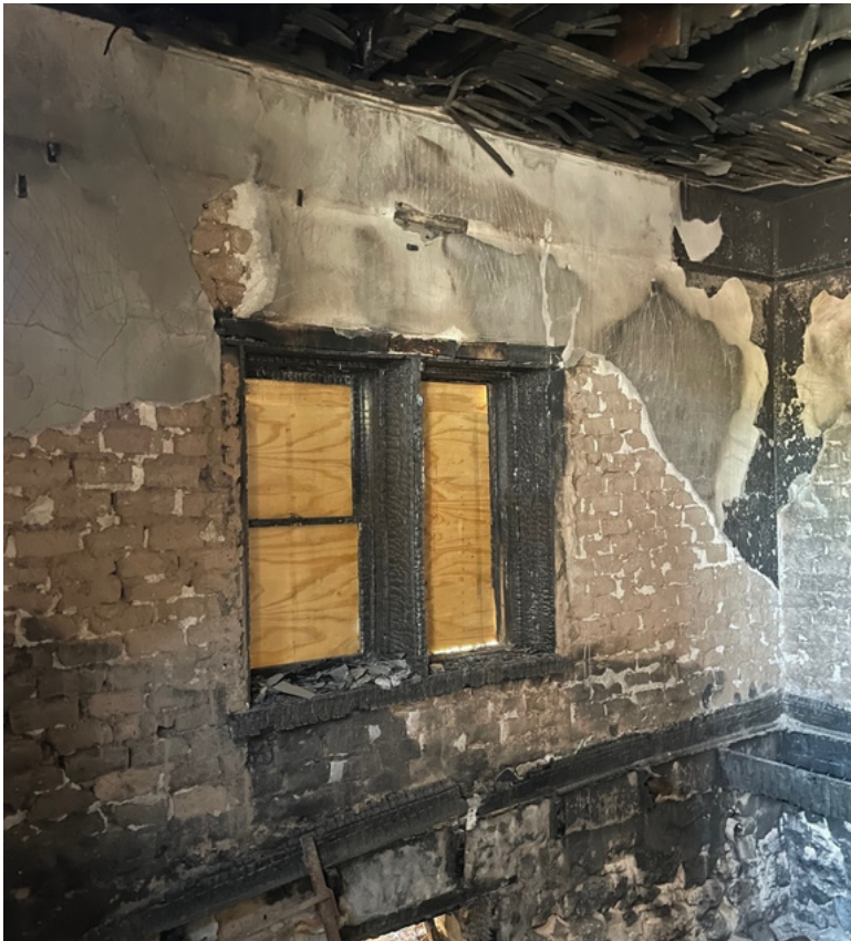
water and fire damage to structural adobe walls
