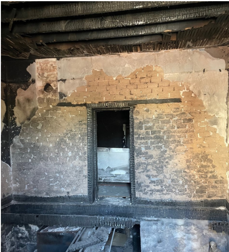
irreparable structural damage to wood and beams
