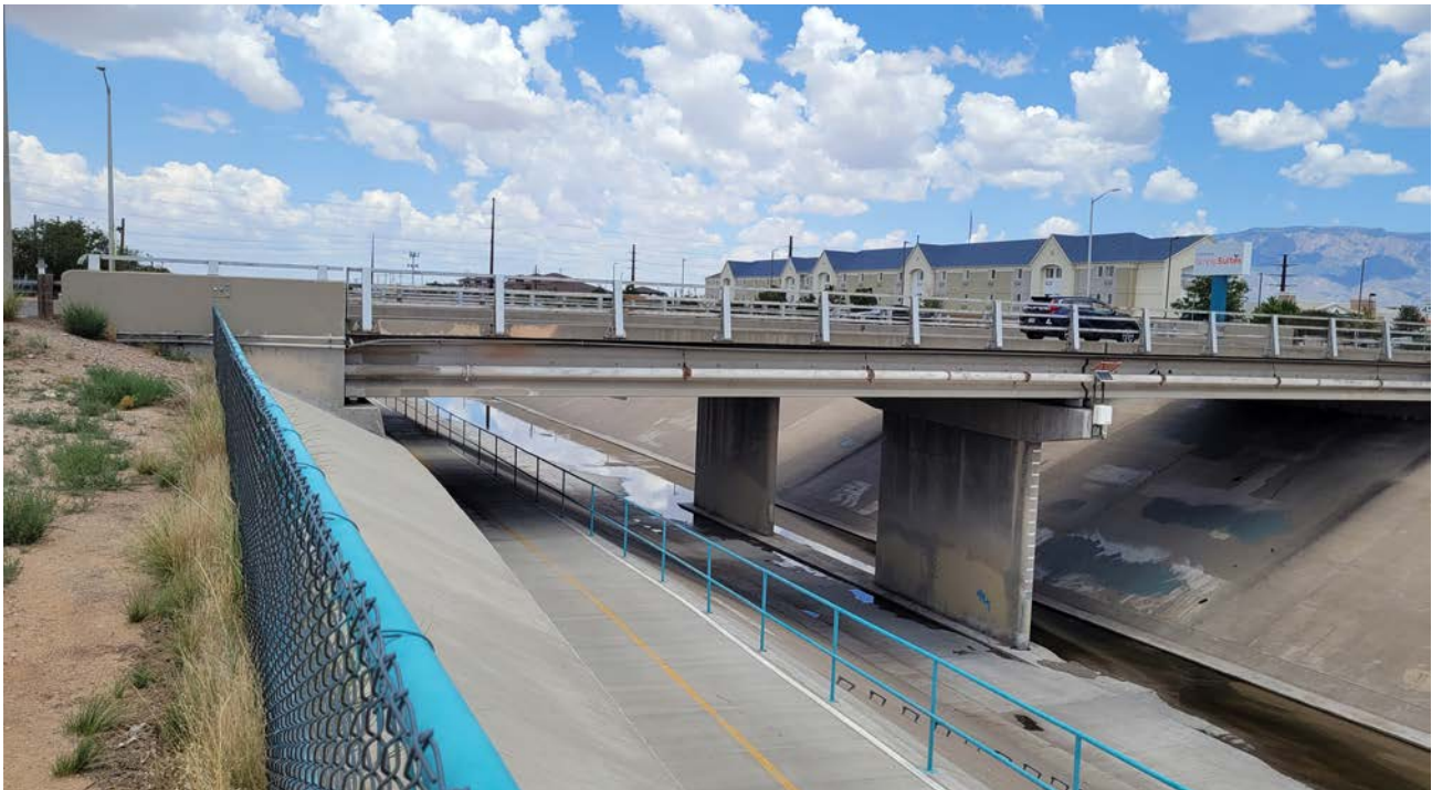
North Diversion Channel Multi-Use Trail.
