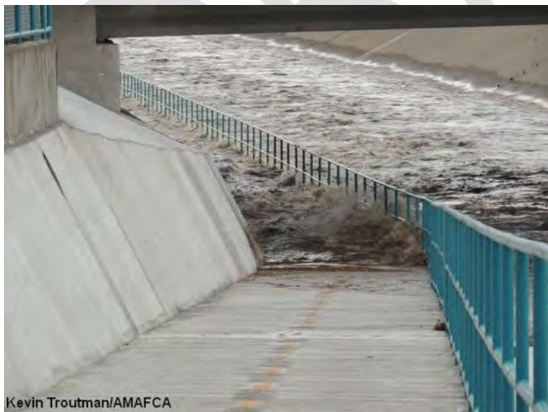
Figure 4-23 Flooding along the Osuna Bike Notch on July 26th, 2013
