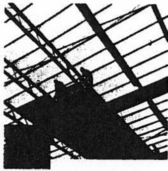
This is a Tectum roof deck going into place.
