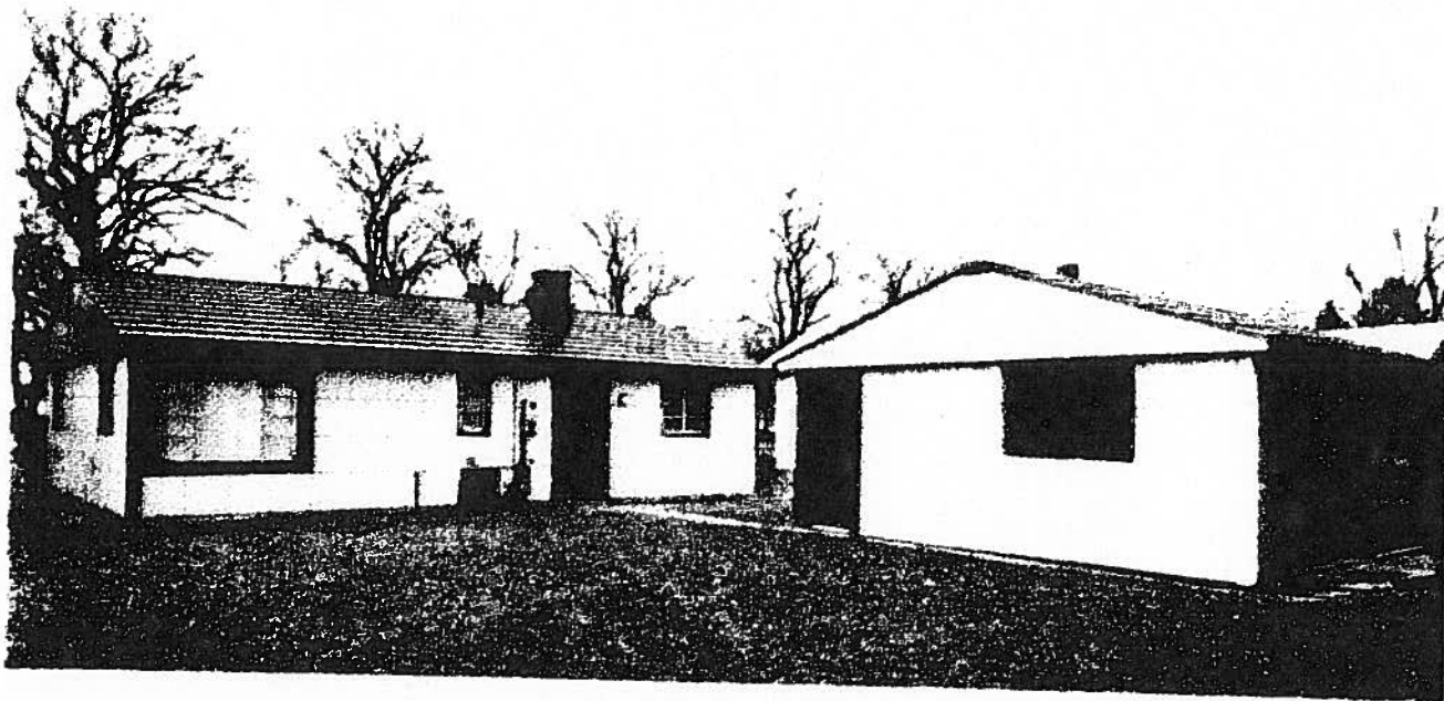
Completed in the spring of 1950, this pre-fabricated, all-metal Lustron House, Porter County, Indiana, was considered by many at the time to be the house of the future. (Beverly Overmeyer, April, 1992)
