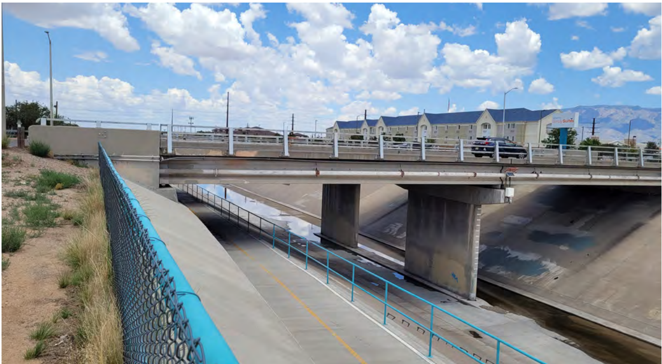
North Diversion Channel Multi-Use Bike Trail.
