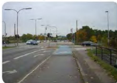
At this unsignalized right turn, the cycle track has dropped to a bike lane with blue coloration and pavement markings through the conflict area.
