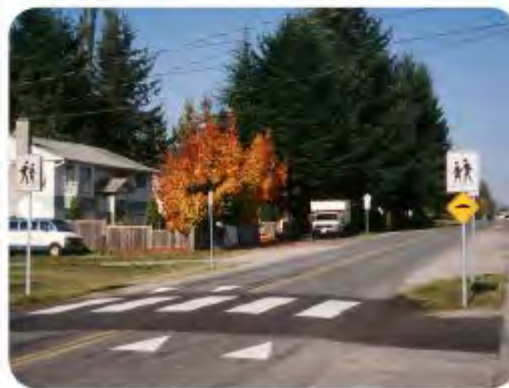
Speed humps are a common traffic calming treatment, which should not be used on emergency routes.
