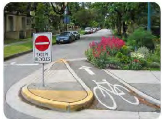
Choker entrances prevent vehicular traffic from turning from a main street onto a traffic-calmed bicycle boulevard.
