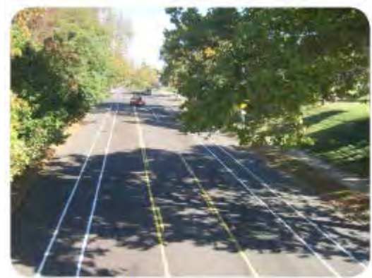
This road was re-stripped to convert four vehicle travel lanes into three travel lanes with bike lanes.
