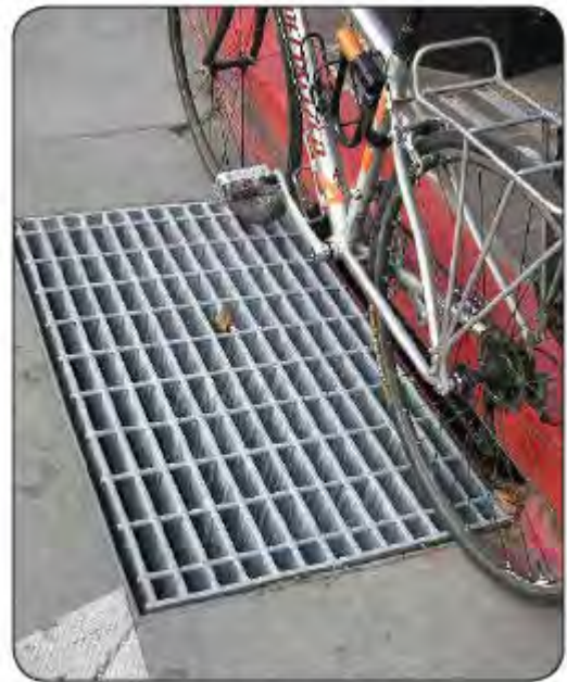
Examples of bicycle-safe drainage grates.
