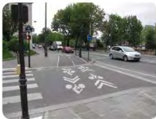
Pavement markings indicate travel direction at a minor roadway crossing on this cycle track in Paris, France.
