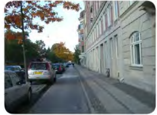
Cycle track with a parking buffer, Copenhagen.
