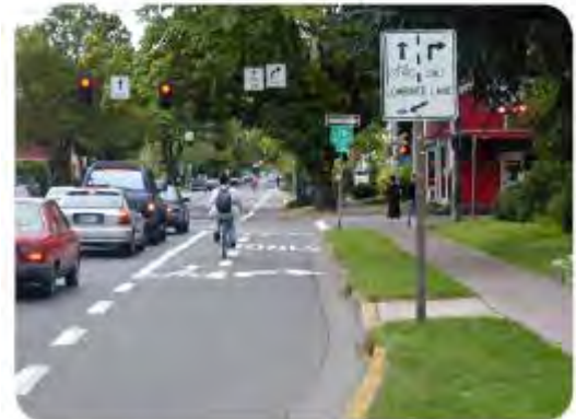
Shared bike-right turn lanes require warning signage as well as pavement markings.
