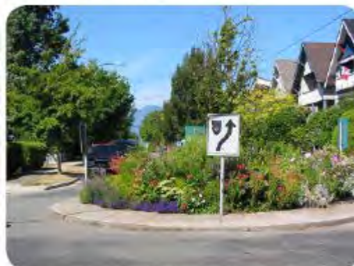
Traffic circles provide an opportunity for landscaping, but visibility should be maintained.
