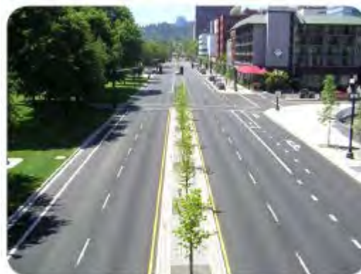
This street in Portland, Oregon previously had 13' lanes, which were narrowed to accommodate bike lanes without removing a lane.
