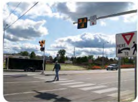
Pedestrian hybrid signal; also called HAWK signals (High-Intensity Activated Crosswalk).
