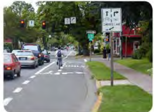
Shared bike-right turn lanes require warning signage as well as pavement markings.
