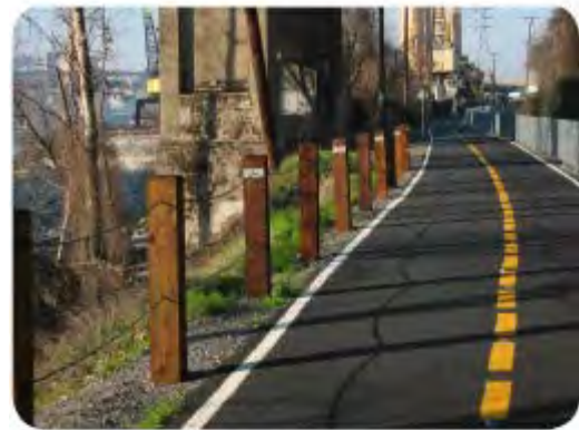
Post and wire fence.
