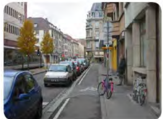
Bicycle markings at a driveway crossing.
