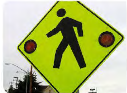
Flashing warning sign.
