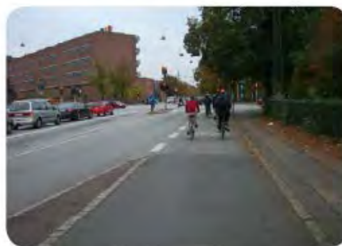
Cycle track dropping to bike lane before an intersection.
