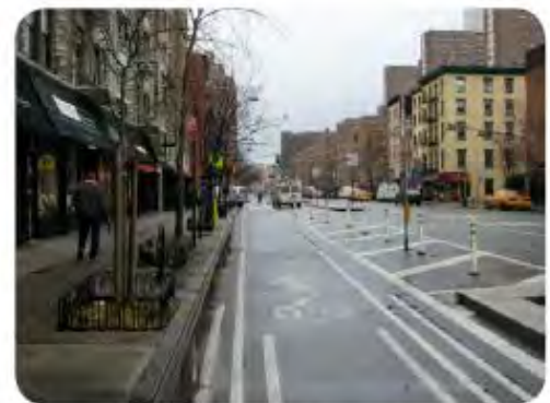
Cycle track with bollard separation, New York City.
