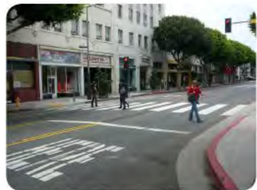
Advance stop bars alert motorists of pedestrians.
