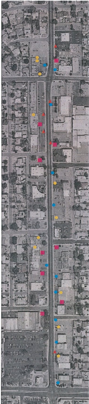
Damaged curb edges
