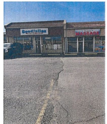
Uneven/cracked parking surfaces
