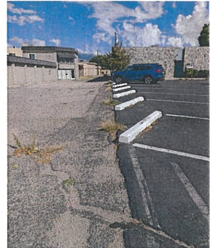
Uneven/cracked parking surfaces
