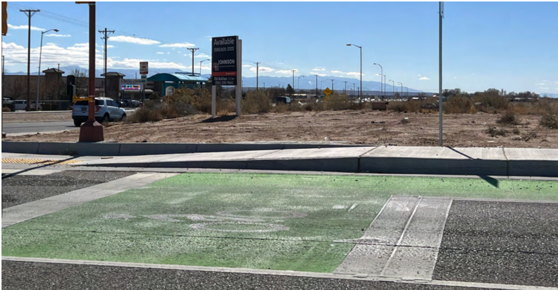
Caption: Bike Lane and Bike Box Located at Coors Blvd. and Tower Rd. Intersection
