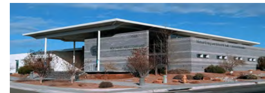
Caption: APD North West Area Substation
