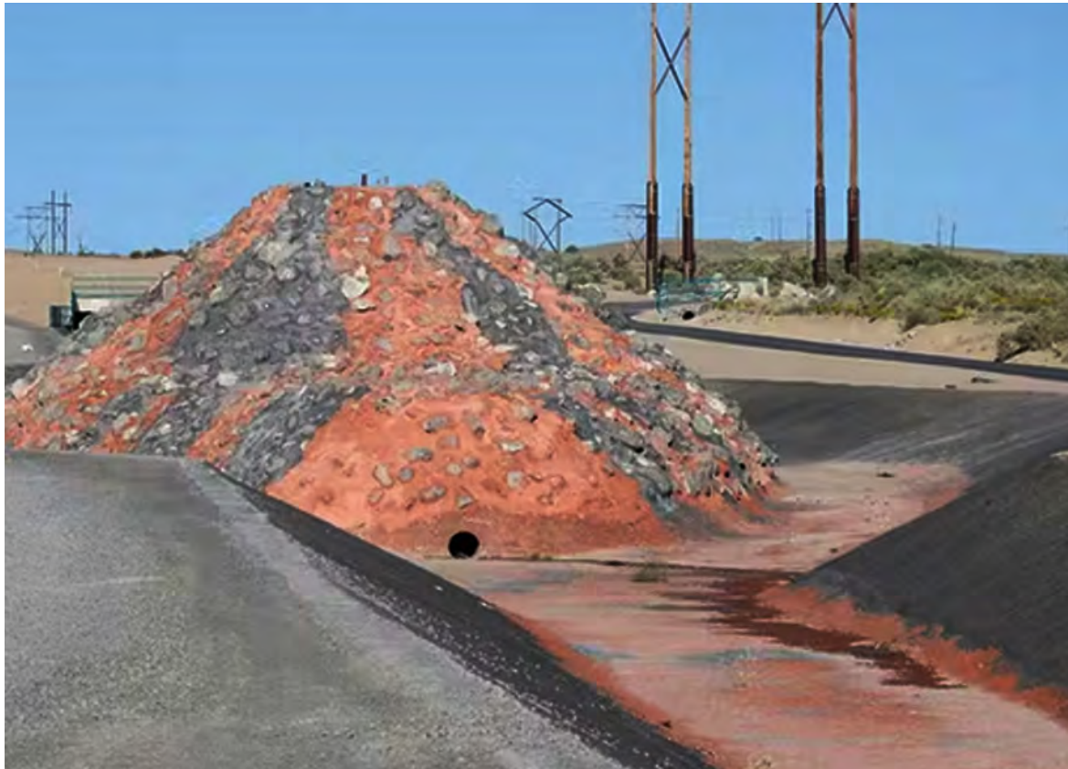
Caption: AMAFCA Drainage ditch Volcano at 98th street and Interstate 40.
