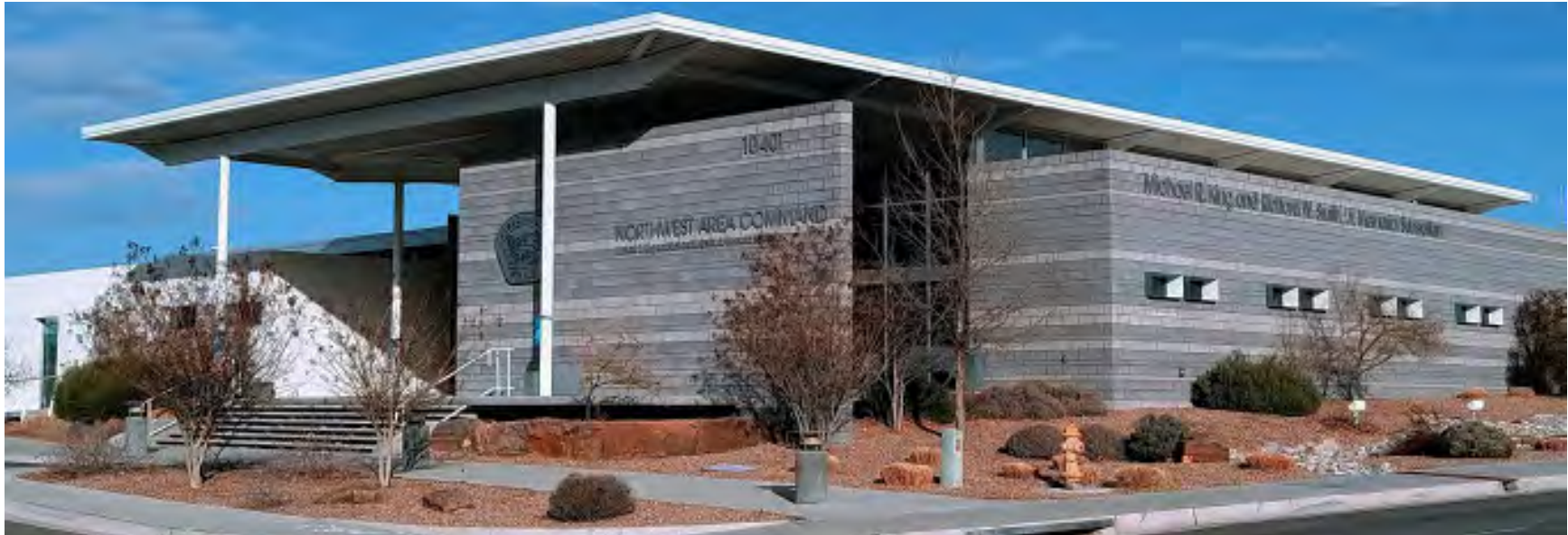
Caption: APD Northwest Command Area Sub-Station
