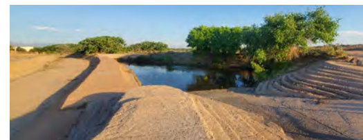
Caption: Mariposa Diversion Canal Pond
