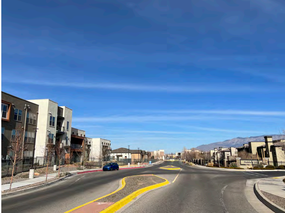
Caption: Mixed Use Development at Coors and Motaño
