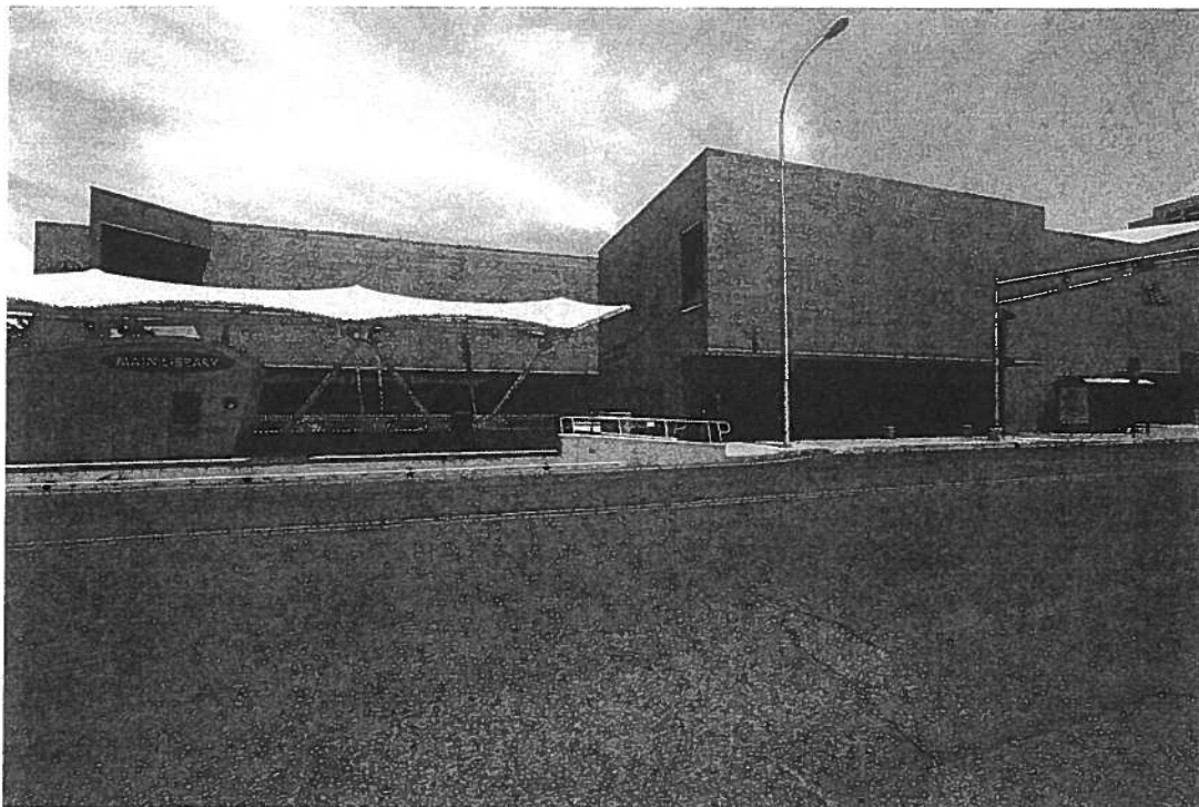
6. South side with ART bus shelter, photographer facing north.
