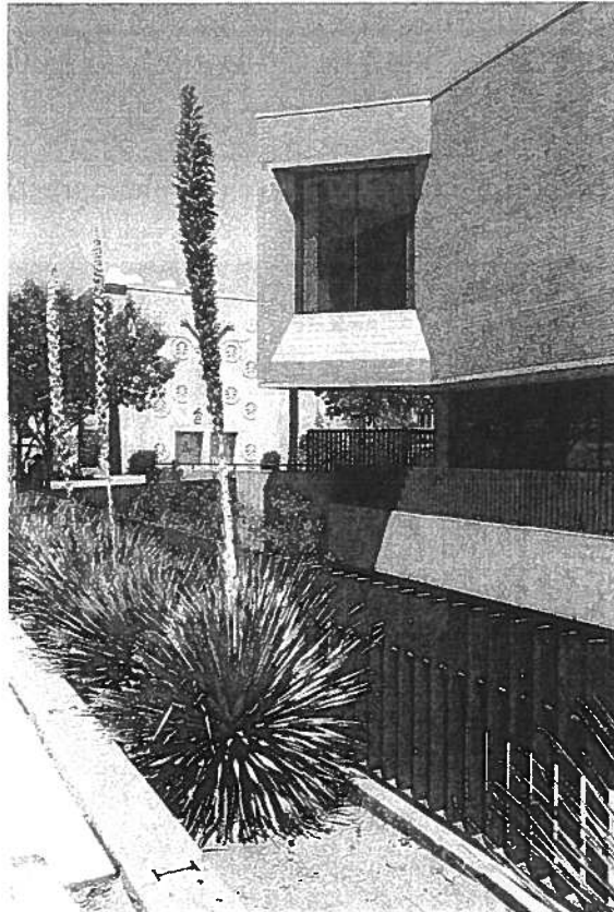
8. Southwest corner, with court and landscaping, photographer facing northwest.
