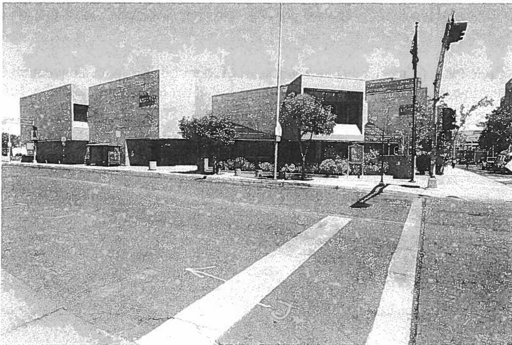
2. South side with glass entrance additions from Copper Avenue, photographer facing northwest.
