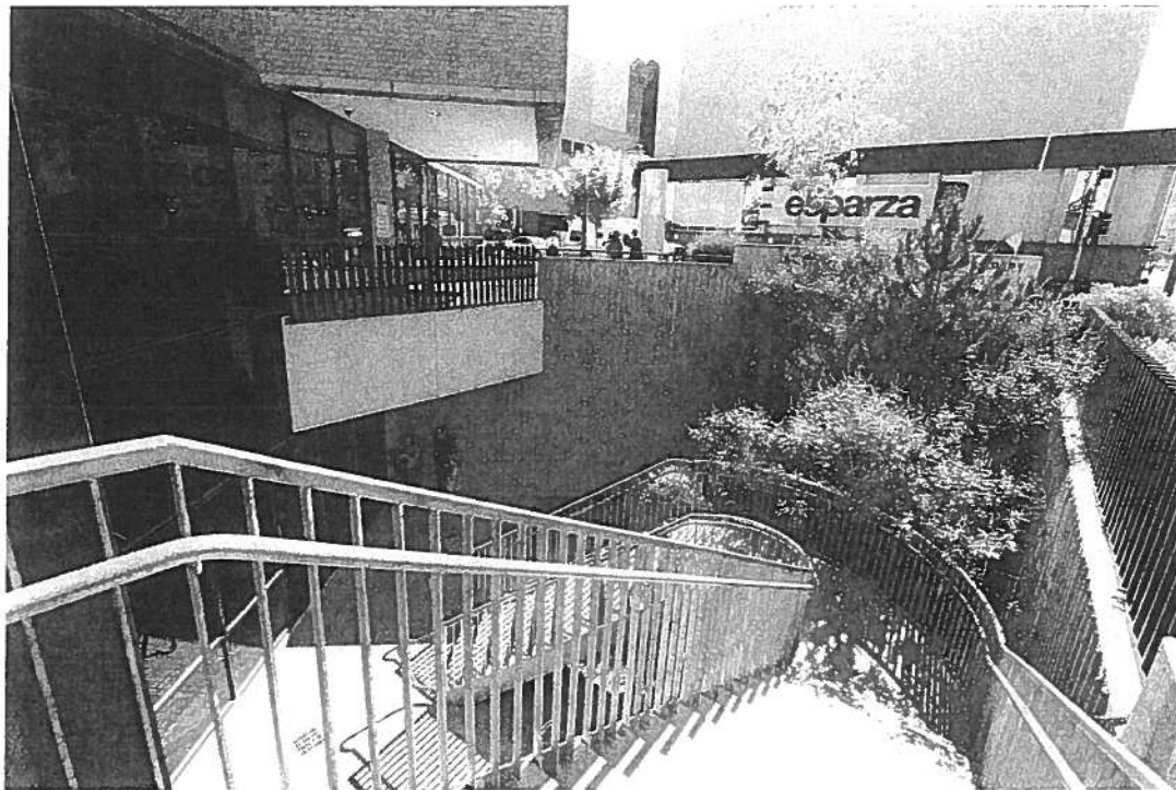
29. Lower level, southeast court, photographer facing east.
