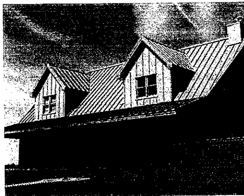
Figure 9: Cool Metal Roofing
