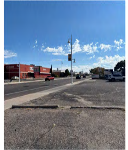
Uneven/cracked parking surface
