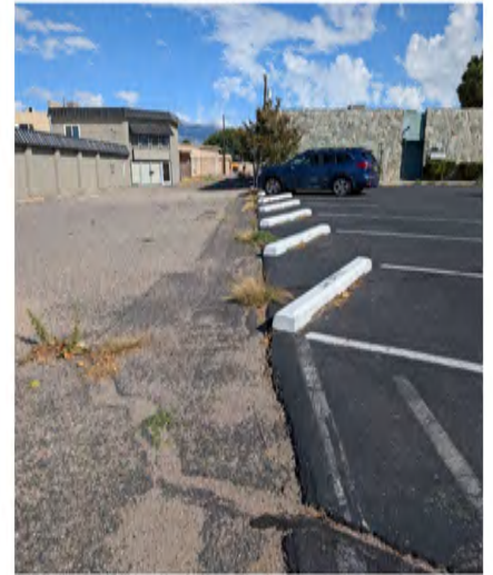
Uneven/cracked parking surfaces
