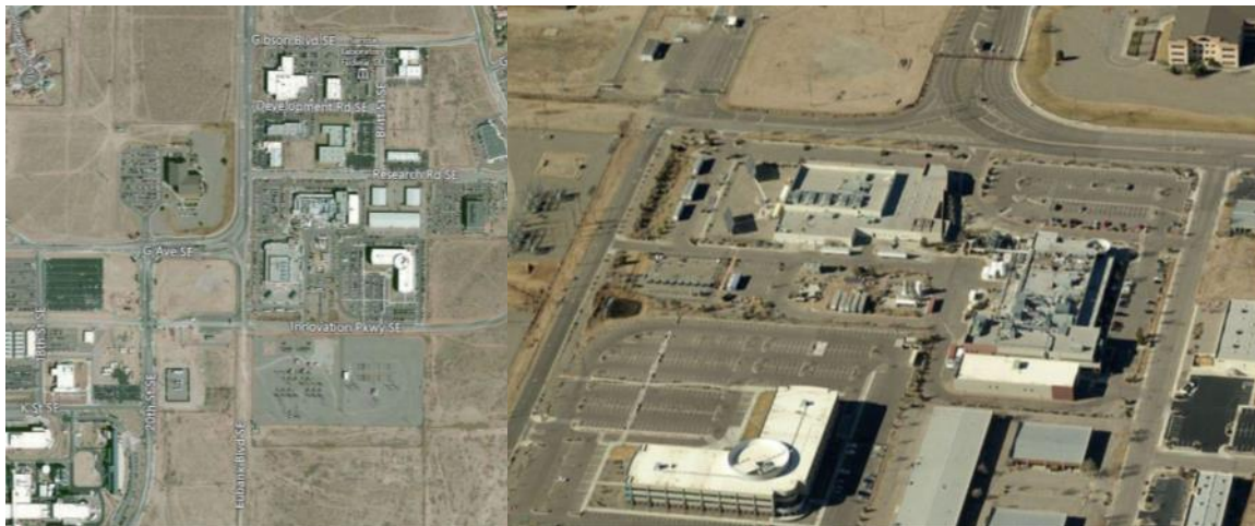
Figure A.2. Schematic view of the current SolAero site. Building 1, shaded in blue, is 84,500 sq. ft. housing a 40,000 sq. ft. cleanroom for compound semiconductor production operations. To the east of Building 1 is 17,000 sq. ft. of Class 10000 cleanroom space for
